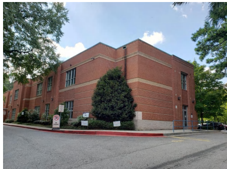
7). Northeast Elevation - Oct 14, 2019
